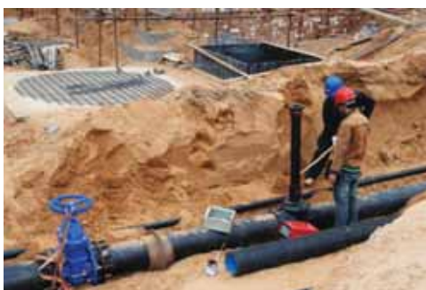
Laying Plant Infrastructure
