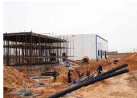
Compressed Air / Nitrogen Station
