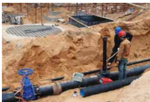
Laying Plant Infrastructure
